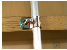
STEP 2: Slide the 3/8 metal clamp over the rod and compress with your fingers. Screw the clamp onto the corner of the top porch.
