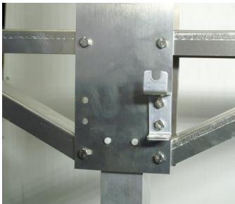
**READ EACH METHOD THOROUGHLY BEFORE PROCEEDING TO DETERMINE WHICH METHOD IS BEST FOR YOUR PARTICULAR HOUSING. IMPORTANT:** Whichever method you choose, orientation of the plate relative to the entrance side of the house is critical. DO NOT position your houses that the entrances face the pole.
