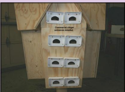
*Here is a possible entrance and no porch scenario with purchased clinger entrances. The front pieces are temporarily attached to the house for clarity. The front pieces can be attached with screws or with hinges once the entire house is painted. This set of entrances do not require a porch.*
