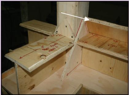
**Countersink, pre-drill and screw the first roof section to the larger gable as illustrated. One screw will hold it in place until the other roof side is attached. Assemble the roof on the opposite side as well.**
