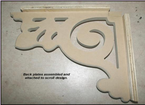
*The completed fretwork can be sanded, primed and painted before attaching it to the martin house later.*
