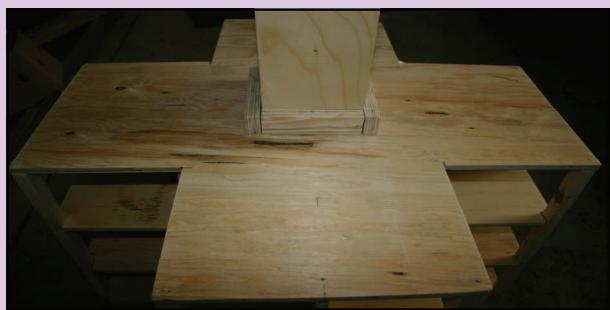
*Pass the first floor 28" x 28" through the post tube and nail it from the top. Be sure the nails enter the bottom cleat shown.*
