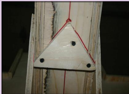
*Install these smaller pieces at the indicated mark using 1 1/4 ' dry wall screws. Angle the screws so they do not protrude inside the post hole section.*
