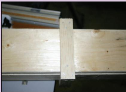
*Nail the pieces to the tube section so they do not pass through the center section. Use 1 1/2" galvanized nails. To interlock the corresponding pieces.*
