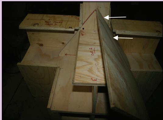
**Fasten the roof section into the upper room roof panel from the side.**
