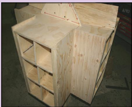
*The image illustrates the proper positioning of the two sides. The sides are flush with the front of the house and bottom floor. Any overlap in the fronts can be removed by sanding.*
