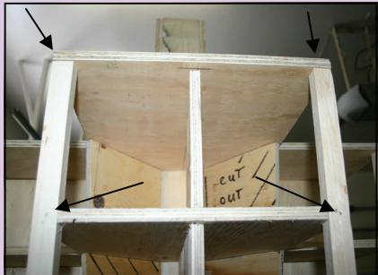
*Nail the braces to the front of each section of the house from the top and bottom as well as to each individual floor with 1" galvanized nails. The previous cut out slots on the second and third floor may be adjusted to accommodate the brace angle.*
