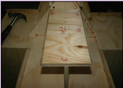
**These pair of roof sections will be attached to the section with the larger roof gables. (larger triangle wood section).**
