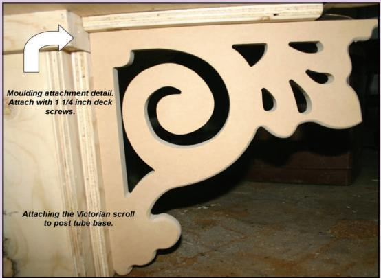
*The fretwork bracket can be added before or after painting the house with eight deck screws. It is easier to mount the house on the pole without the fretwork.*
