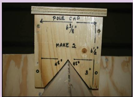
***Mark and cut out two opposite side pieces as illustrated and angle cut the bottom to accommodate the roof sections. The roof cap length can be adjusted to suit your individual pole and pulley configuration. A good test is to take a piece of pole and pulley assembly and test the cap for proper fit.***
