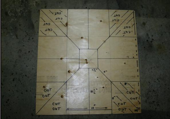
*After cutting the first panel 28"x28", mark out the panel by drawing diagonals from corner to corner. Measure the post tube section or trace the tube section (5 1/4" square) onto the plywood next and continue laying out the pattern accordingly to accommodate the room sizes. The hashed section 8" x 8" will be cut out.*
