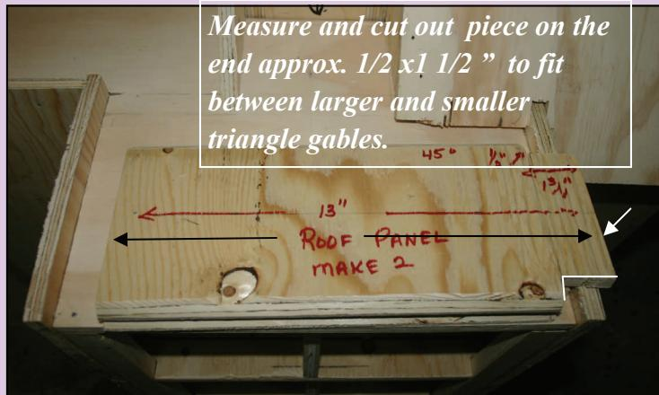
**The illustration indicates how the roof, the larger roof gable, and the roof section are finally assembled.**
