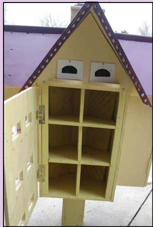
*As an option the front doors may also be left in one piece and attached with four deck screws or installed so that there are two door sections without hinges. In this photo, the bottom and top pieces have been cut and the bottom portion is secured with two 3 inch non mortised (bi-fold) hinges. They are positioned 3" from the top and bottom of the door. The upper door section is held in place with two screws for easy access and cleanout.*
