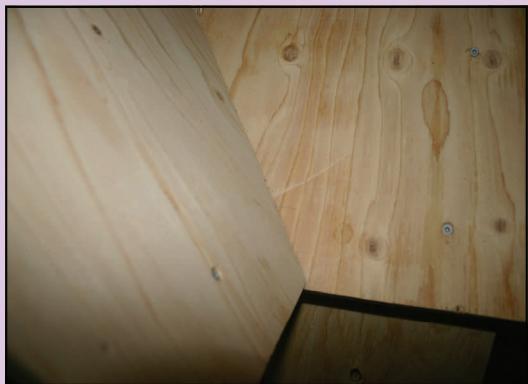
**Close up detail of the roof sections. If these sections do not align, scribe and angle cut the roof section until it meets the other correctly.**
