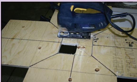
*Cut the post holes using a jig saw in all floors ensuring that they are all the same. Very Important! Check your post tube to ensure that the floors will pass through it.*
