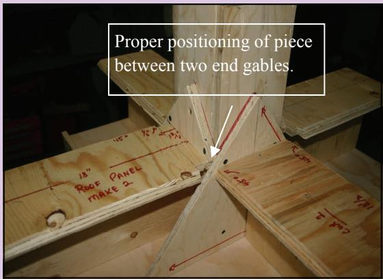
**Nail all the roof sections and the dividers to the roof gables and floors.**
