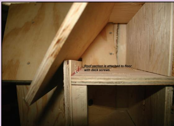
**Fasten the roof section to the side wall into the upper floor section from each side with deck screws.**
