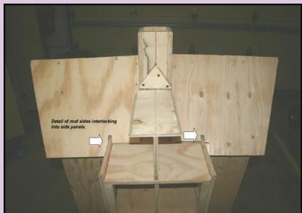
**The two larger gable opposite roof sides have now been assembled and fit neatly into the wall sides. Proceed to the next smaller roof sections and assemble accordingly.**
