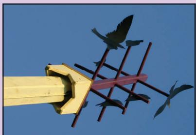
***Attach the post cap to the end of the post with 4 deck screws . Similarly, attach mast head with silhouettes to post cap with 4 deck screws .***
