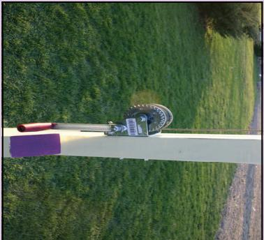
***Install pole base and attach winch to post with two 3/8 " x 4" bolts ,washers and lock nuts. Attach 40 feet of 3/8" galvanized aircraft cable to the winch.***
