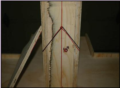
*Using the larger triangular section, mark the walls on the center post on all four sides.*
