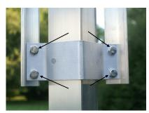
Step 3: Remove the 4 bolts that attach the bottom hub brackets. Keep the nuts and bolts because to reattach the new hub brackets.
