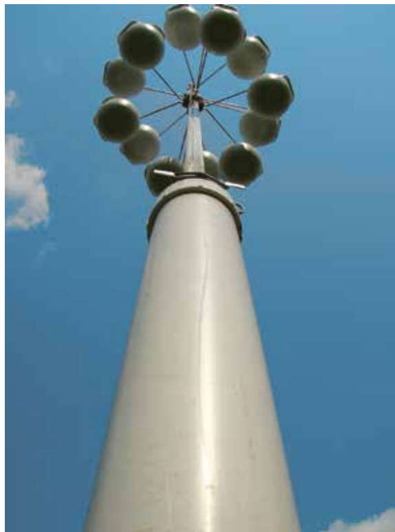
Above: What the raccoon or snake sees — a long, formidable expanse of PVC pipe.
